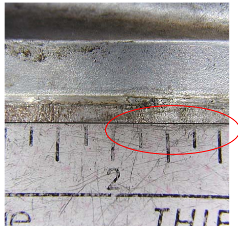
This close-up photograph shows where a crack was identified on unit 2. The crack was verified using UT in place and ET when removed. Best viewed at 200% zoom.
